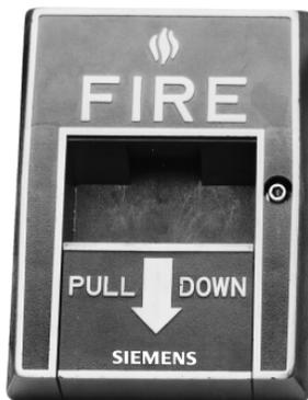
Pull down the bar on the fire alarm station to activate the alarm.
